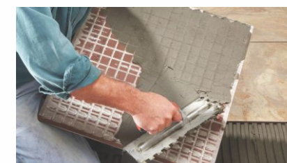
2. Cement laying on Tile
