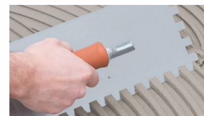
1. Cement laying on Floor
