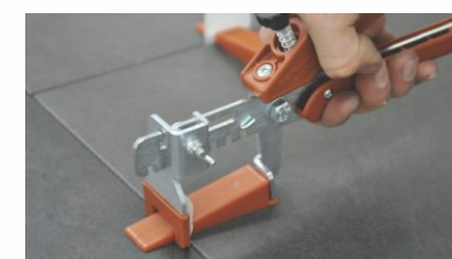
4. Levelling Wedges
