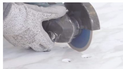
2. Cut with Diamond Blade Angle Grinder
