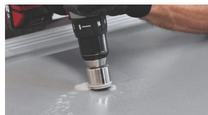
1. Round Cut with Diamond Blade Drill
