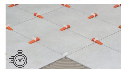
5. After Levelling Process leave it for 8-10 hrs.
