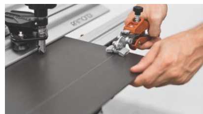
2. Cutting of Tile
